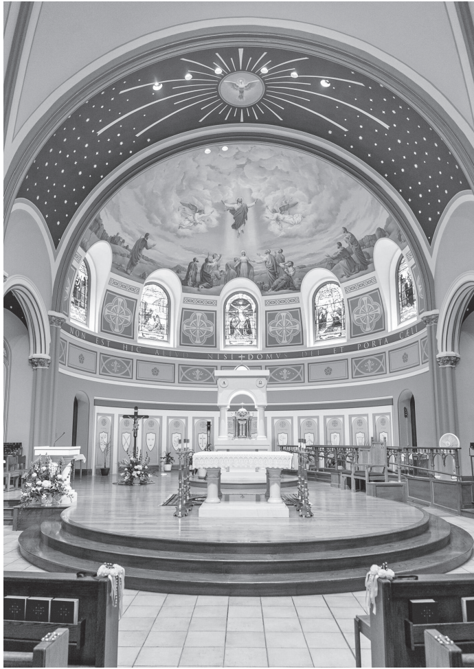
Figure 6. Closeup of restored sanctuary.
